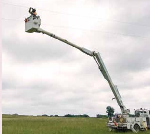
Twin Valley Lineman **SETH STRASSER** repairs a ravin on Highway 160. A ravin is when a strand of the aluminum conductor breaks. This affects the electrical performance of the conductor and can affect the tensile strength. Line maintenance and repairs such as this are common at Twin Valley to insure system reliability for our members.
