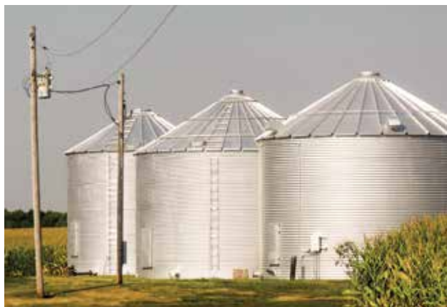
Building a structure too close to overhead power lines can create an electric shock danger during and after construction.
